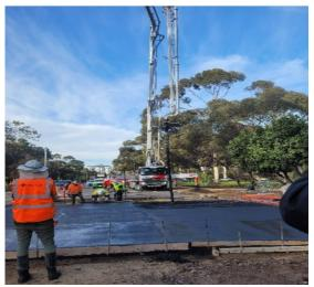
Construction of a signalised raised crossing, which connects the Park Lands trail on both sides of Hutt Road crossing is 50% completed, along with the road works on the southbound section of Hutt Road.
